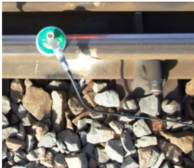
Negative Lug Attached to Welder's Magnetic Clamp
