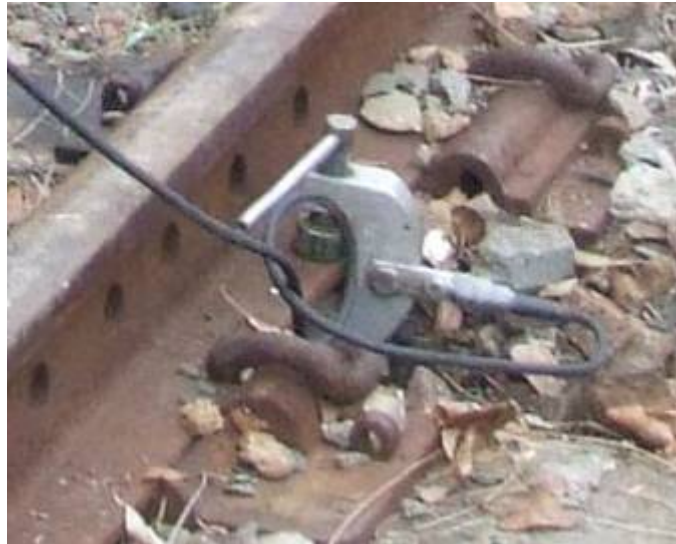
Negative Lug Attached to Pfisterer Rail Clamp on Rusty Rail
