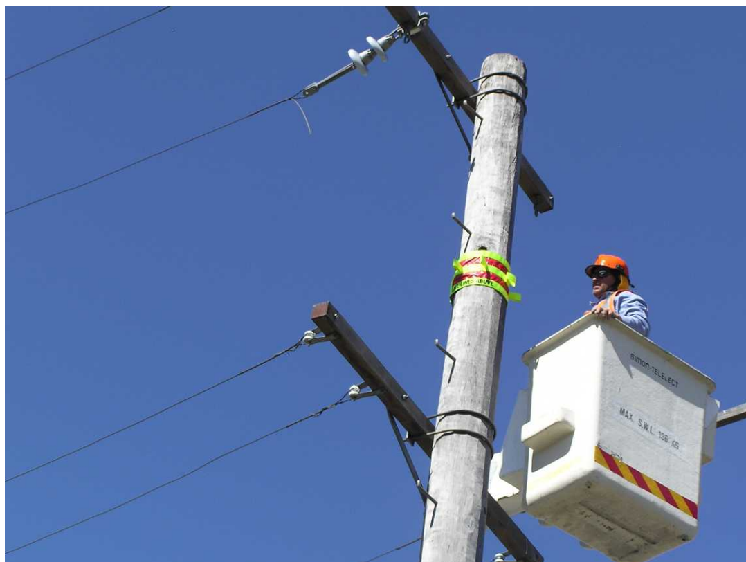
Figure 3 Applying the pole marker from EWP
