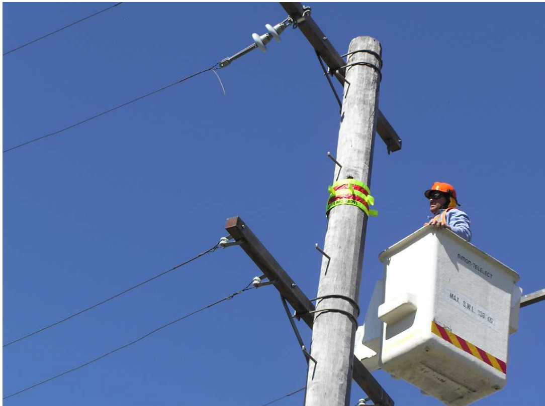
Figure 3 Applying the pole marker from EWP
