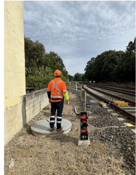
Image 4: View of Down direction Lookout at 141.074 KM (Next to D1 Signal)
