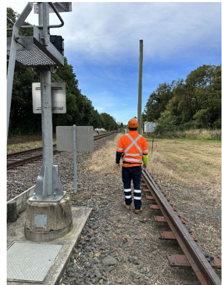
Image 6: View of Down direction Lookout at 141.197 KM (Next to BE 7 Signal)
