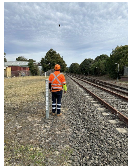
Image 2: View of Down direction Lookout at 140.920 KM (Next to 140.920KM Post)
