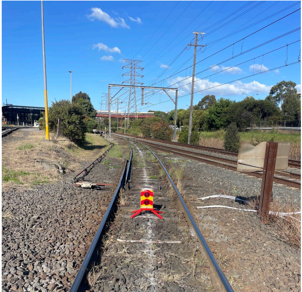
Image 3: Worksite Protection Marker placed clear of 531 Points ( 531 points clipped and locked by Bluescope Road Control)
