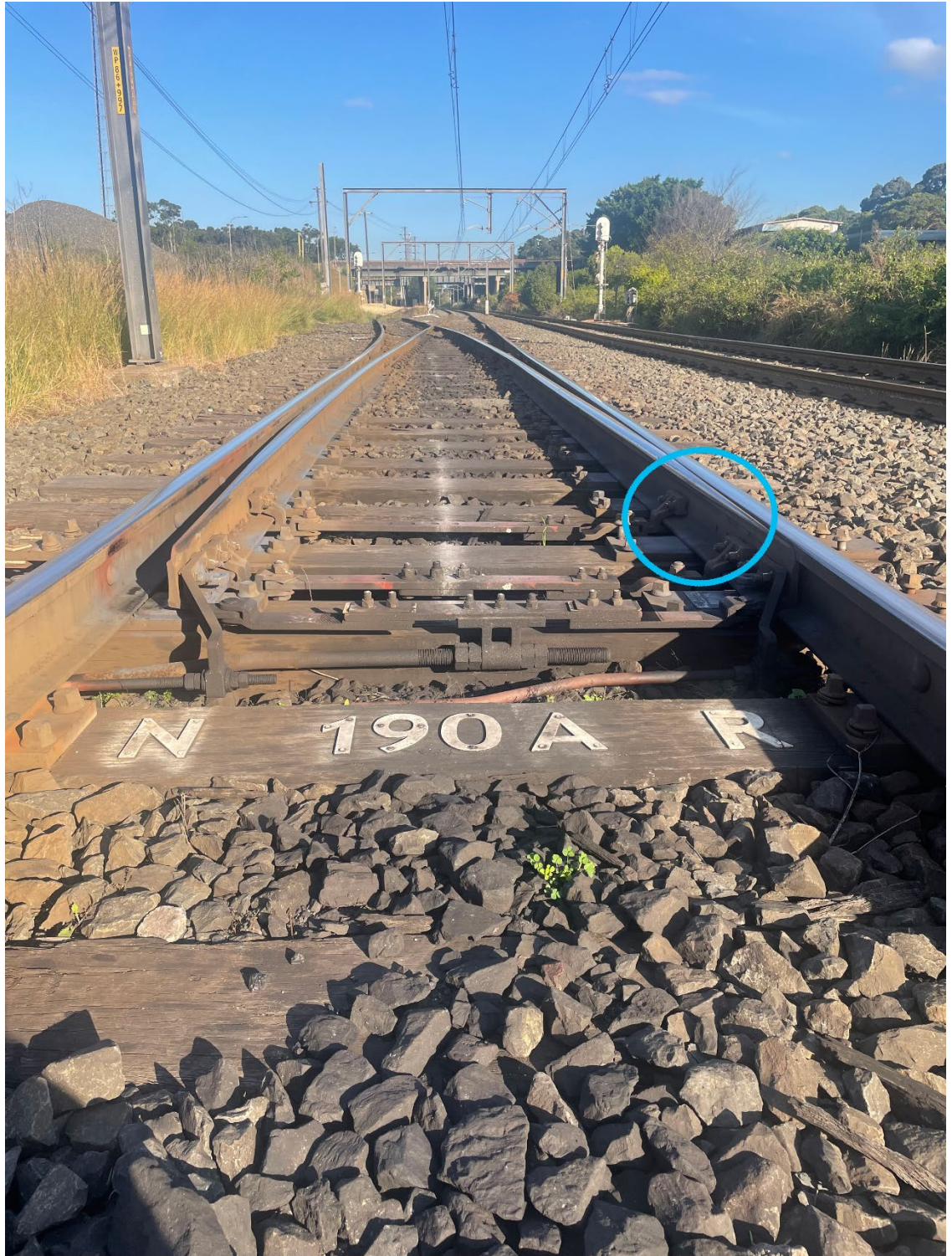
Image 1: Wollongong Side TOA Limits 190 Points (Point Clip position circled)
