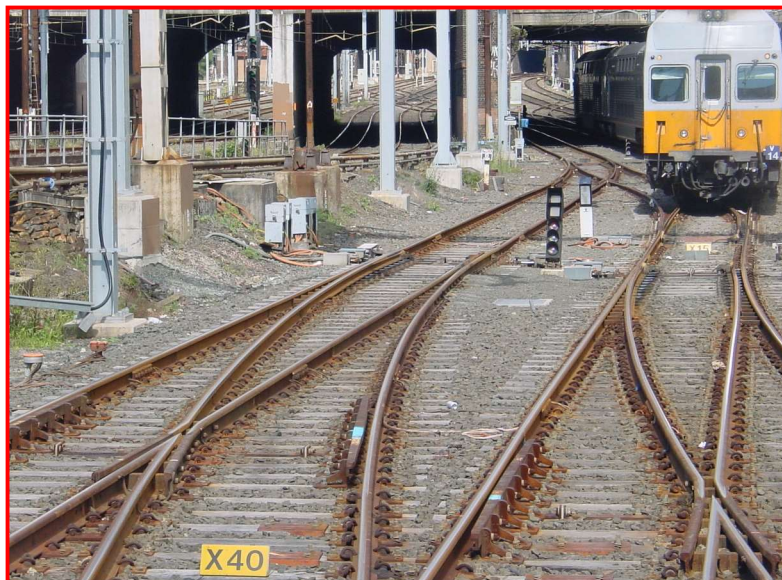
DUE TO THE CLOSE PROXIMITY OF ROADS IN SYDNEY YARD THERE ARE MANY SPEED BOARDS PLACED BETWEEN THE RAILS AS SHOWN
