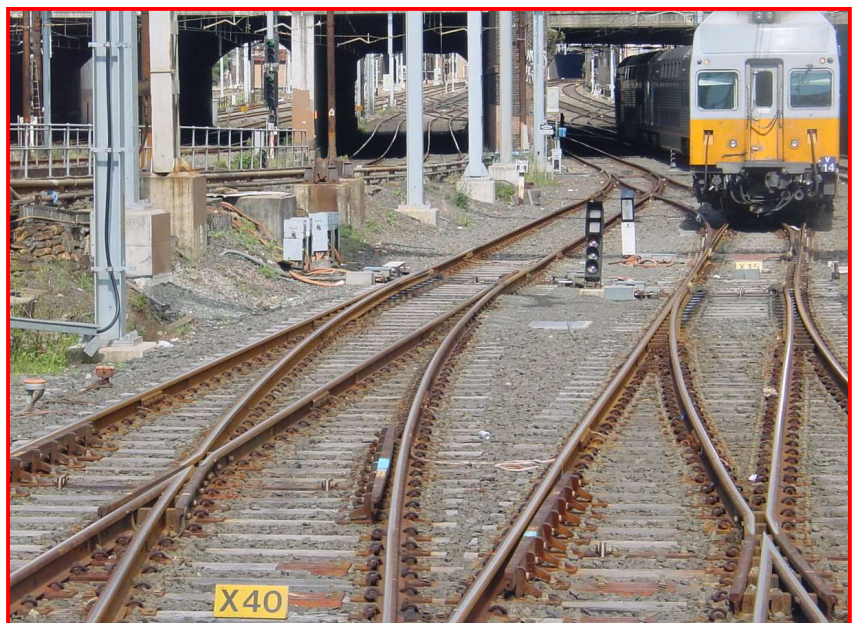
DUE TO THE CLOSE PROXIMITY OF ROADS IN SYDNEY YARD THERE ARE MANY SPEED BOARDS PLACED BETWEEN THE RAILS AS SHOWN
