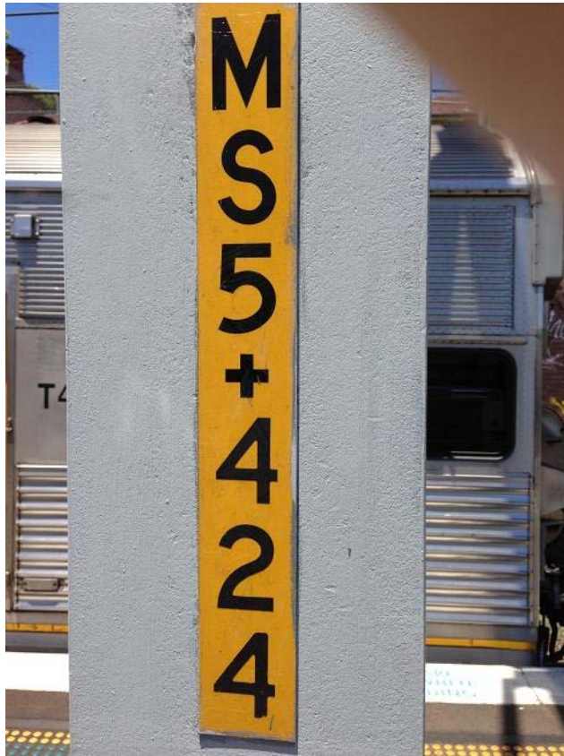
Figure 6 – Example of a OHW structure number label
