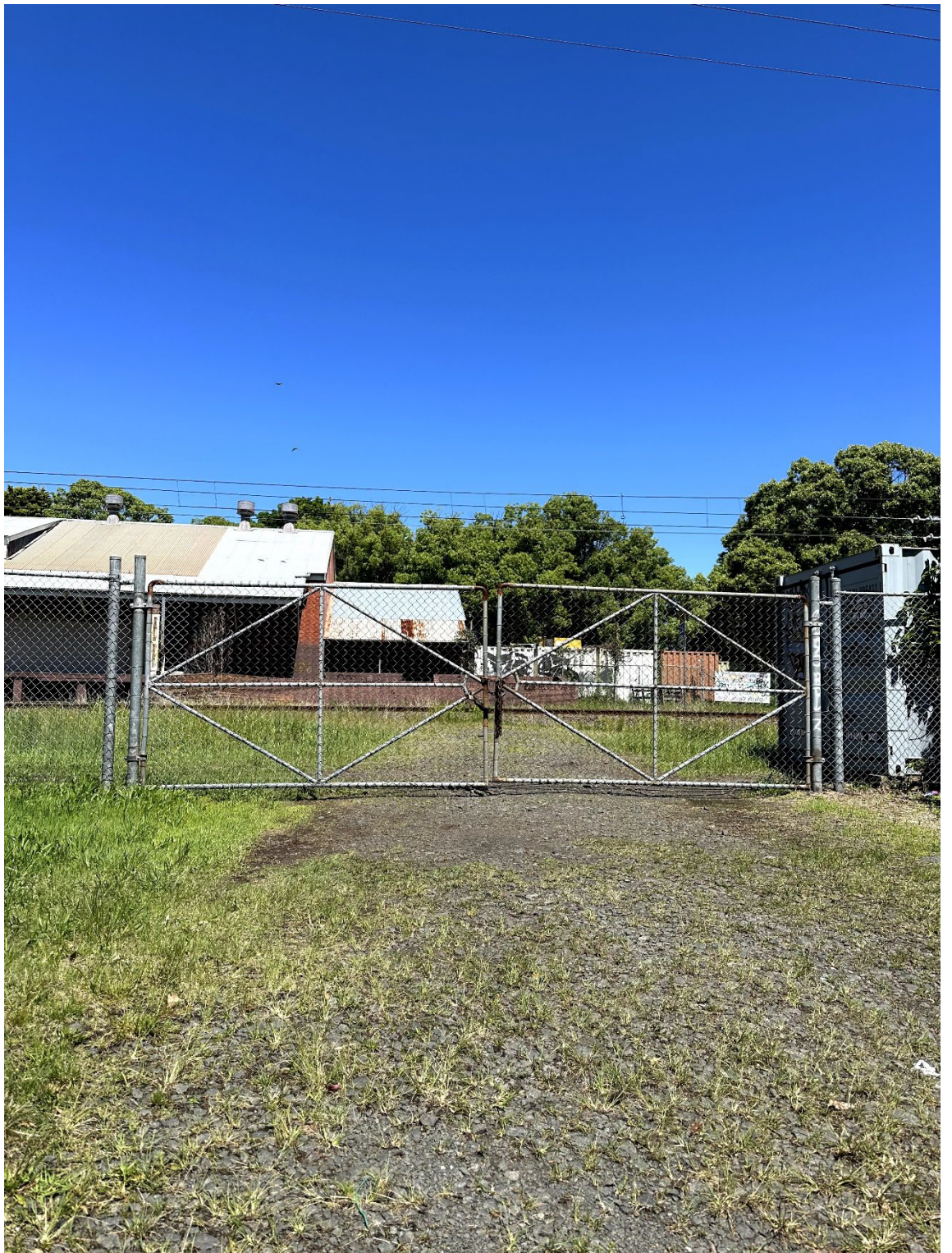
Image 5: Access Gate 100 102.940 D on the Down side. Double Gate along Burroo Street Albion Park Rail
