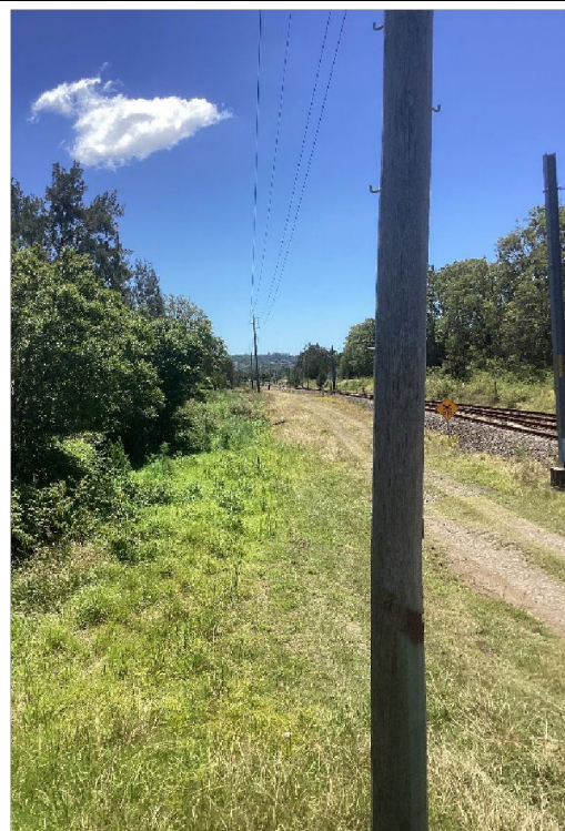
Image 2. Lookouts View: Wollongong Side of Dapto Station facing Wollongong
