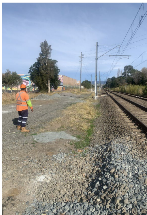
Image 5. Lookouts view Albion Park side of Dapto Station facing Albion Park
