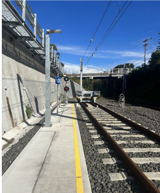
Image 5: Berry Side TOA Limits – End of Terminal Line Kiama Down Siding
