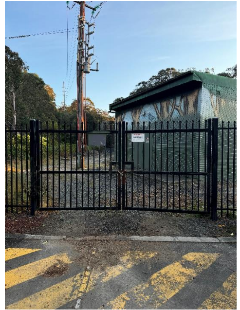
Image 2: Access gate 100 46.168 U to Handsignaller location at 46.250 KM (Rail access road off Old Sta RD)
