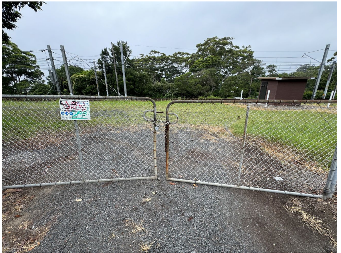
Image 5: Access Gate 100 68.376 at Austinmer on the Up side. Double Gate in the middle Railway Ave Austinmer
