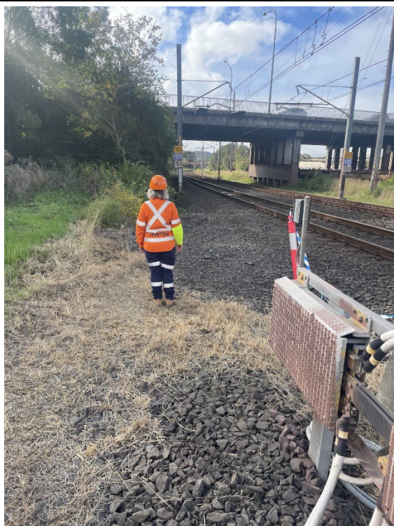
Image 1: Wollongong Side of worksite facing Wollongong (Near WG 1017 U)
