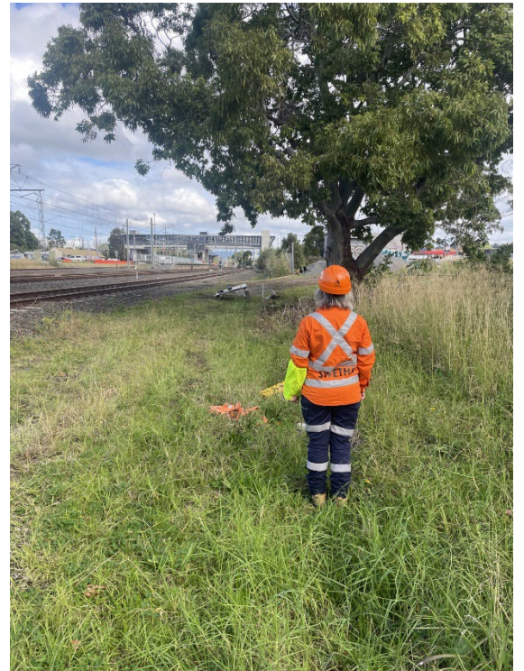
Image 4: Lookouts view (Adjacent to B frame) Facing Dapto
