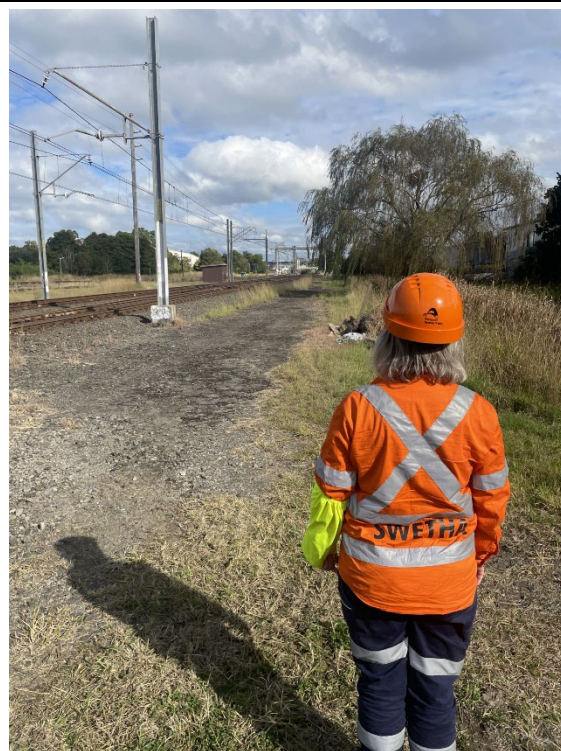
Image 2: Wollongong end of the worksite facing Dapto
