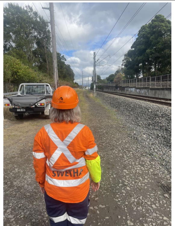
Image 6: Lookouts view Dapto end of the worksite facing Wollongong
