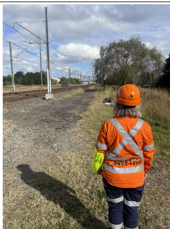
Image 2: Wollongong end of the worksite facing Dapto
