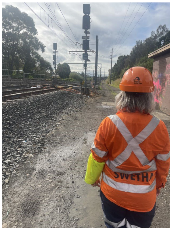
Image 5: Lookouts view Dapto end of the worksite facing Dapto
