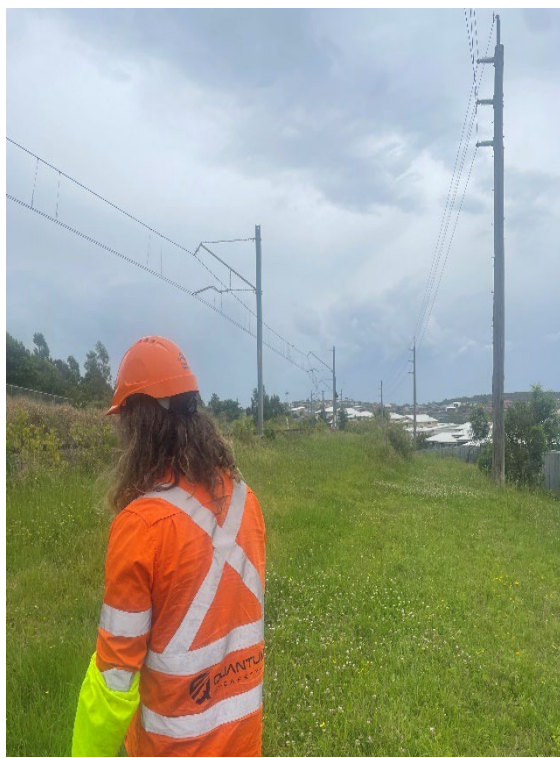
Image 1: Additional Lookout - Wollongong side of worksite
