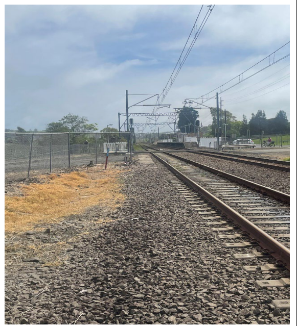
Image 8: Lookouts View Kiama Side of Worksite facing Wollongong
