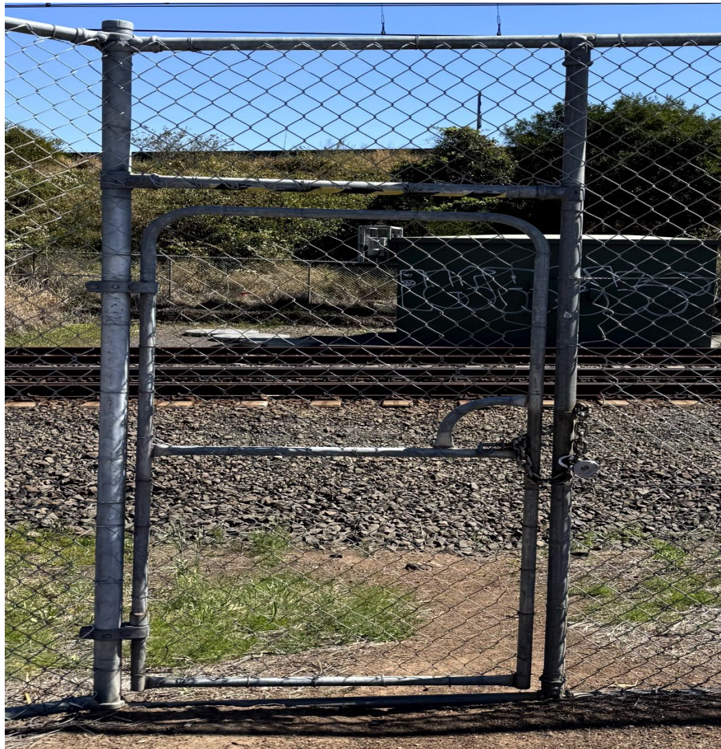
Image 1: Access gate at the end of Piper Road. (adjacent to 51 Points)
