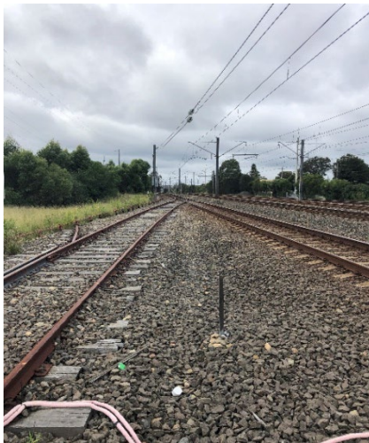
Image 1: View of Down direction Lookout at 46.562 KM 6 foot.
