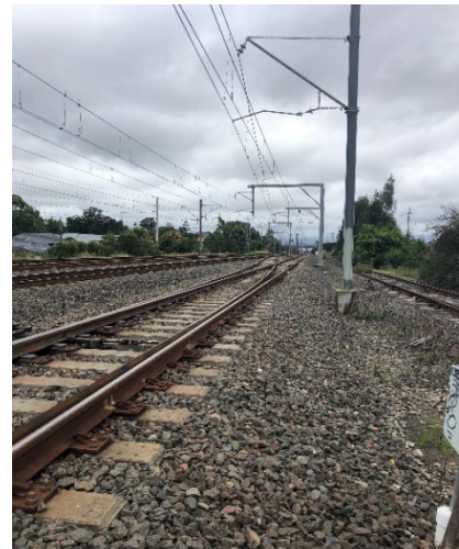
Image 2: View of Up direction Lookout at 46.581 KM 6 foot
