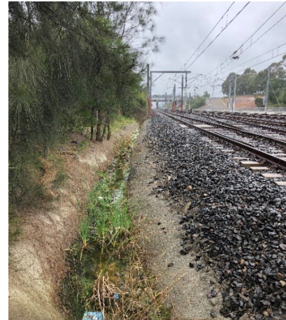
Image 2: View of th Down direction Lookout at 47.189 KM Up cess.
