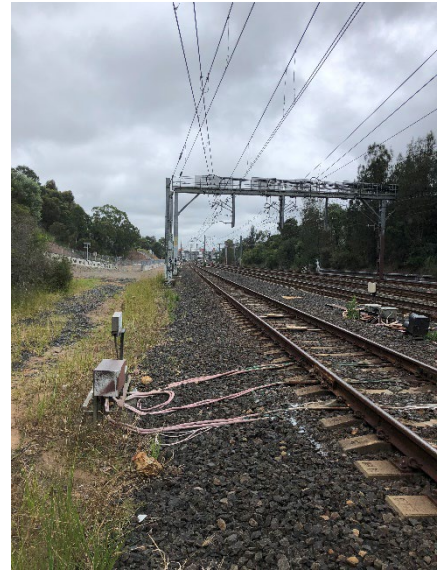
Image 4: View of Up direction Lookout at 47.015 KM Down cess.
