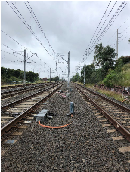
Image 3: View of Down direction Lookout at 46.948 KM 6 foot.
