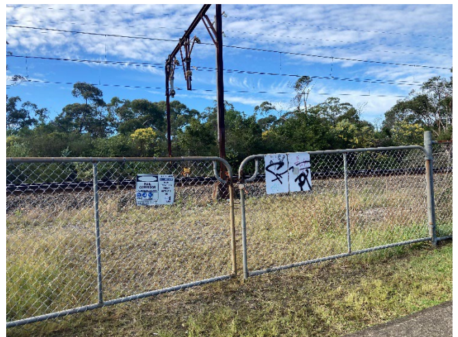
Image 2: Sensor access using access gate N00 40.424 D
