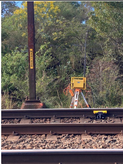
Image 1: Transmitter and sensor installation location
