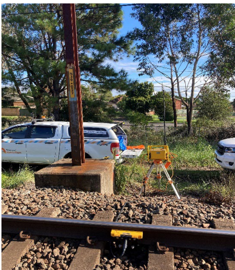
Image 1: Transmitter and sensor installation location
