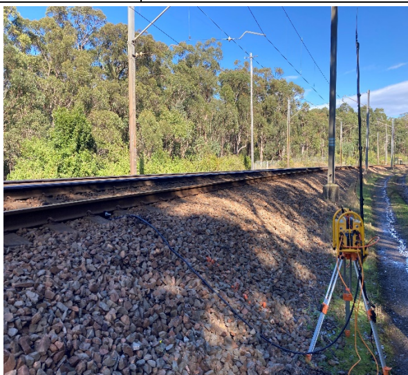
Image 1: Transmitter and sensor installation location
