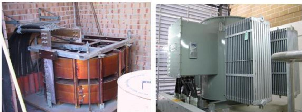
Figure 3 – Examples of air and enclosed negative reactors
