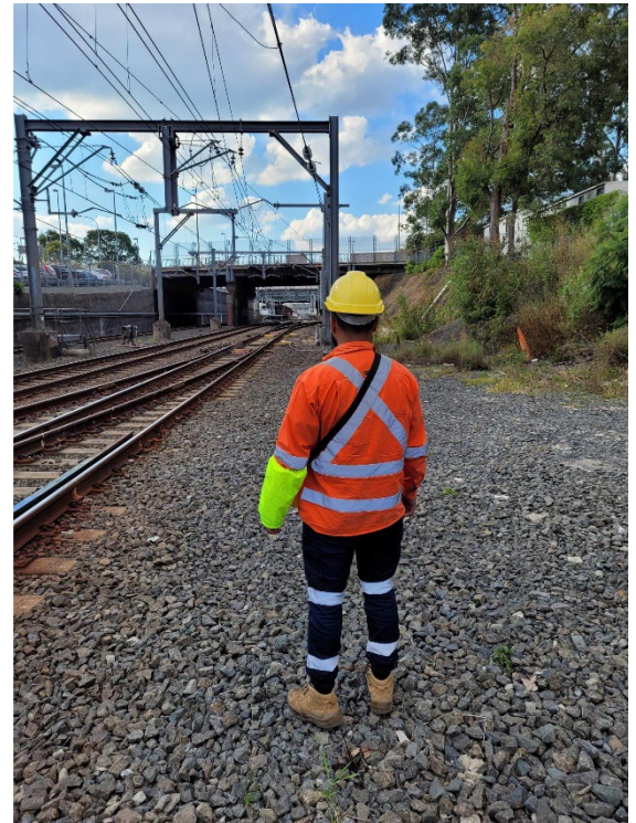
Image 8: Lookout in Up Cess for approaching rail traffic from the Up direction.
