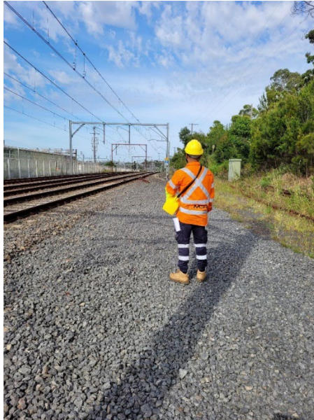
Image 3: Lookout in Down Cess near 574 points looking for approaching rail traffic from the Down direction
