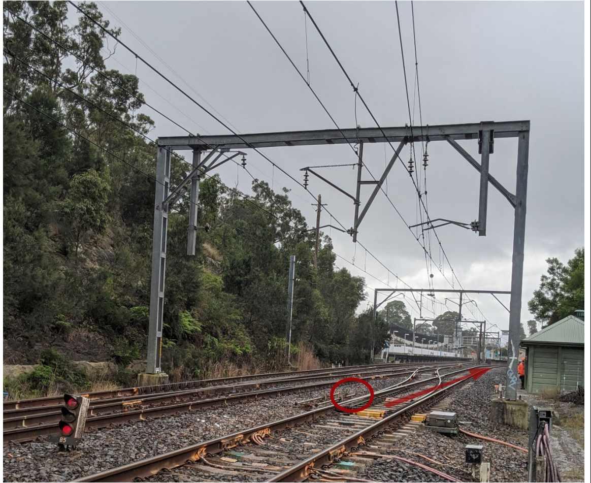
Image 4: B5 at stop and 52 points secured preventing access into the worksite
