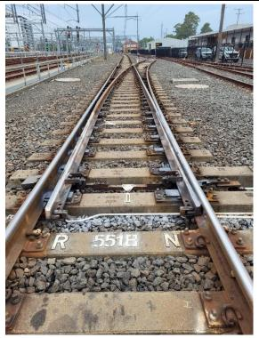
Image 6: (Live adjacent line): View of 551B points in the normal position from **Down Relief** leading into worksite. These points are to be clipped and locked in the **normal** position to prevent entry into the worksite.
