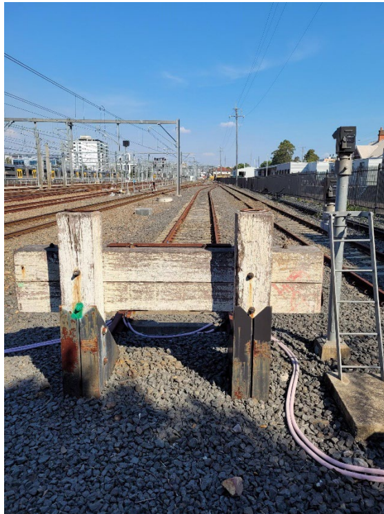
Image 1: View of buffer stop at Country End of Terminal Line for No. 1 Down siding
