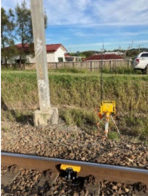
Image 1: Transmitter and sensor installation location
