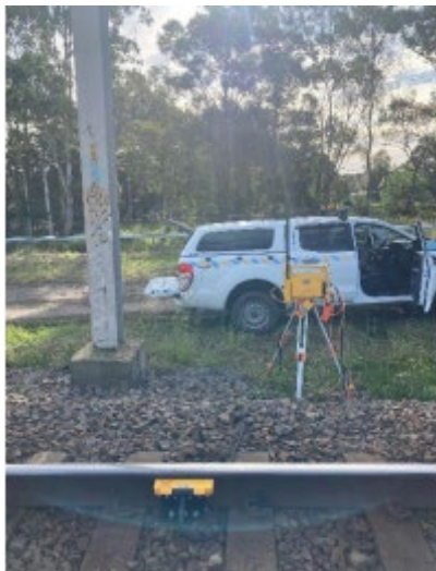
Image 1: Transmitter and sensor installation location
