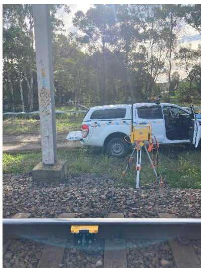
Image 1: Transmitter and sensor installation location
