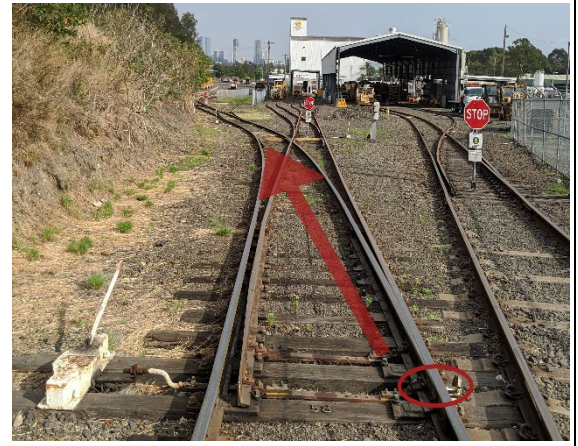
Image 2: 58 points clipped and locked
