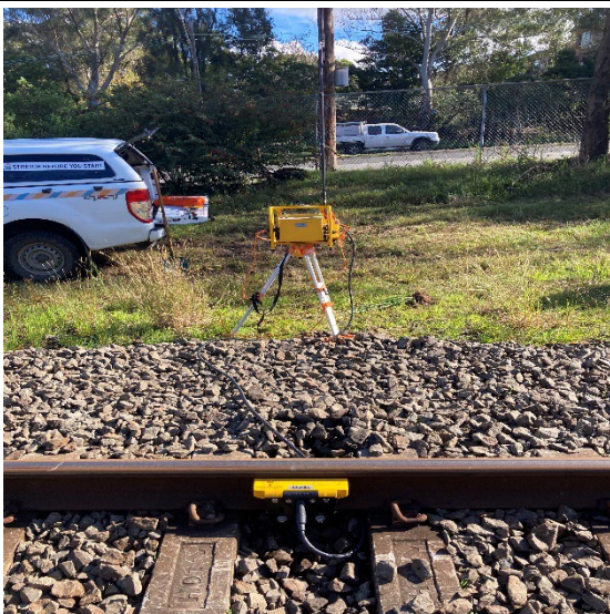
Image 1: Transmitter and sensor installation location
