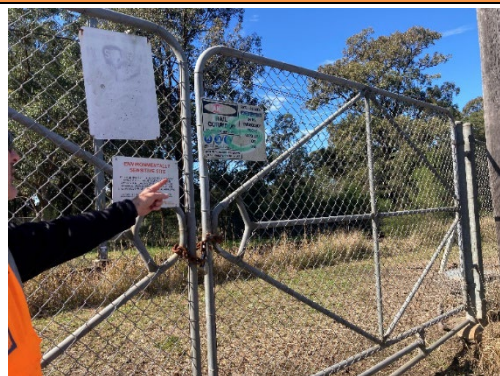
Image 2: Sensor access using access gate M17 51.260 D
