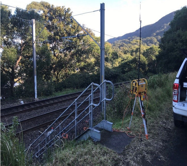
Image 1: Transmitter and sensor installation location
