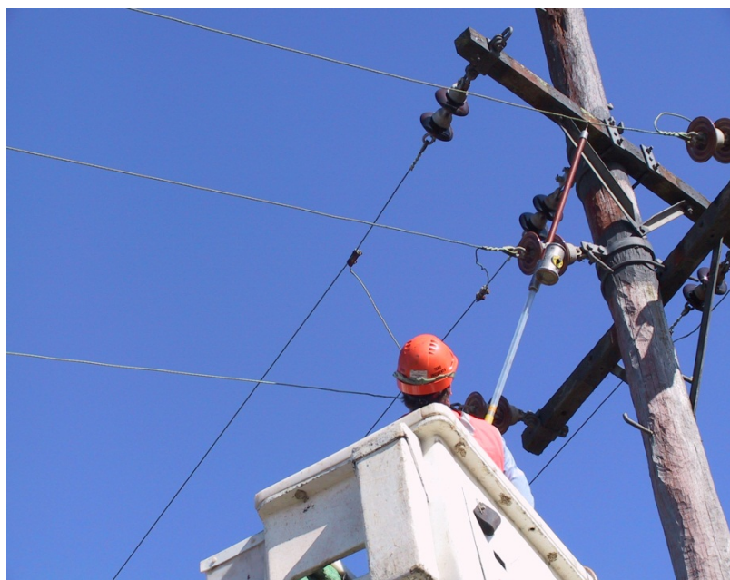
Figure 2 – Testing with high voltage detector
