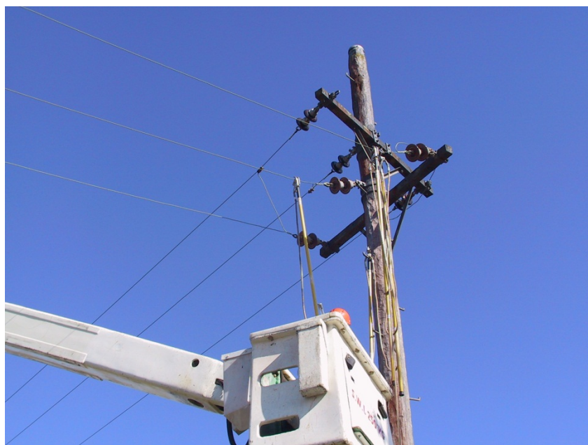
Figure 3 – Application of earths
