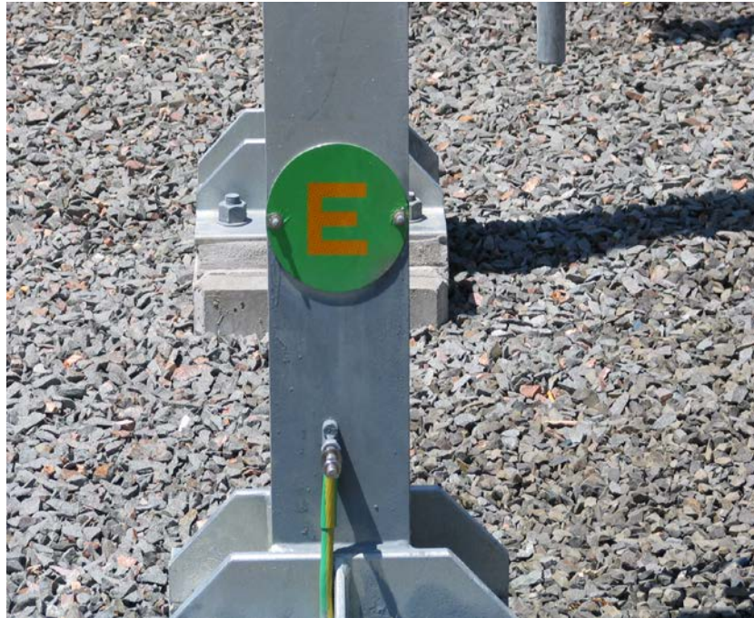
Figure 11 – Typical Substation Earthing disc and Earthing Point
