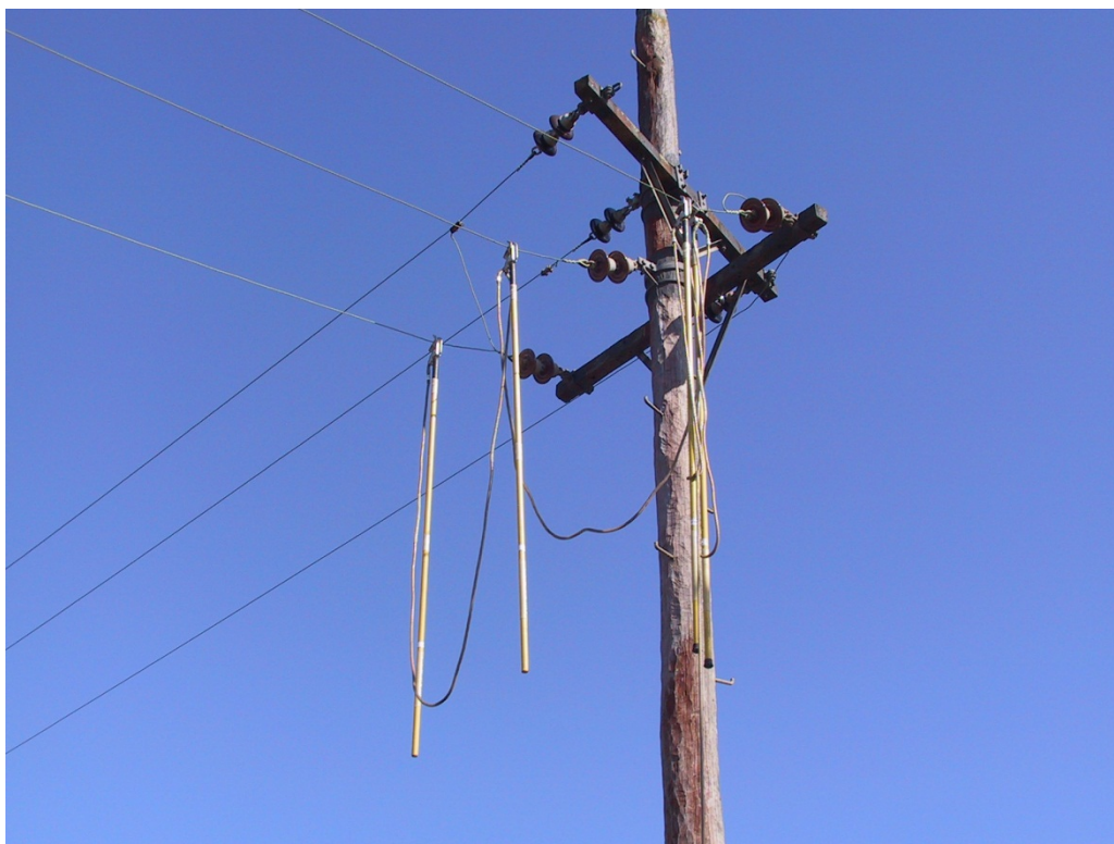
Figure 5 – Earthed aerial conductors
