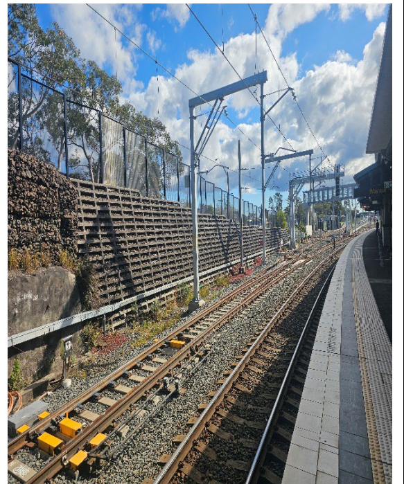
Image 2: View towards city, entry into UP Yard
