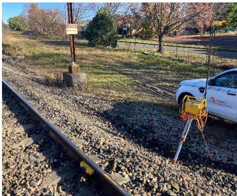
Image 1: Transmitter and sensor installation location
