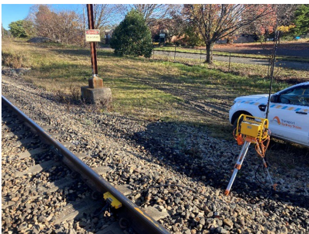
Image 1: Transmitter and sensor installation location
