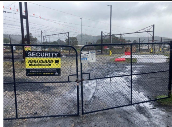
Image 2: Sensor access using access gate W00 153.037 U
