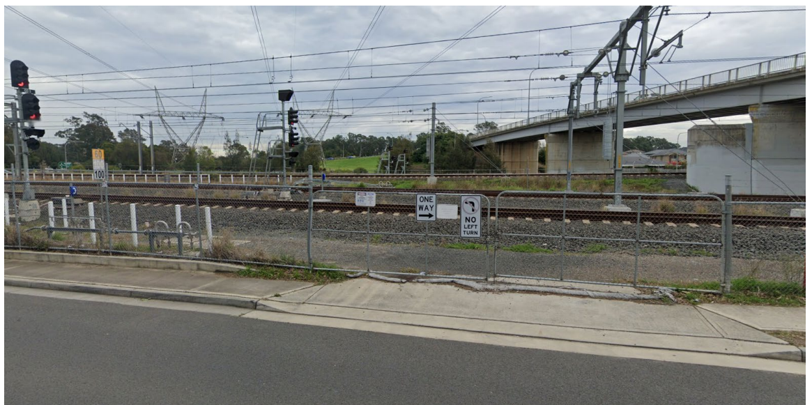
Image 3: access gate M25 32.191 D
