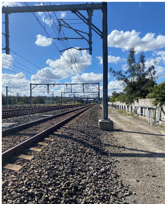
Image 1 View of worksite towards Casula station
