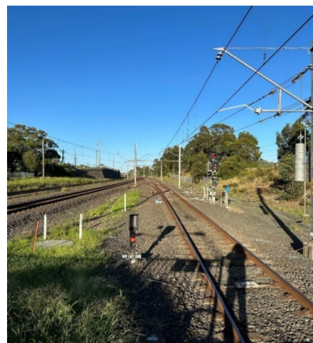
Image 4: View of worksite towards Carramar station
