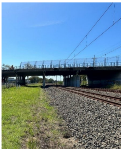
Image 3: View of worksite towards Leightonfield station
