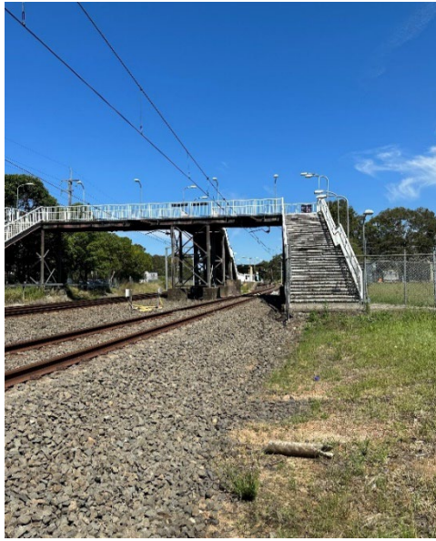
Image 3: View of city side of Villawood Station
