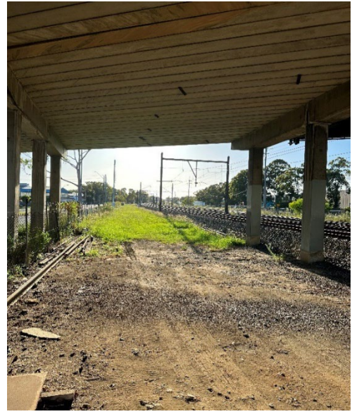
Image 4: View towards Leightonfield Station
