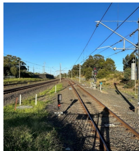
Image 4: View of worksite towards Carramar station
