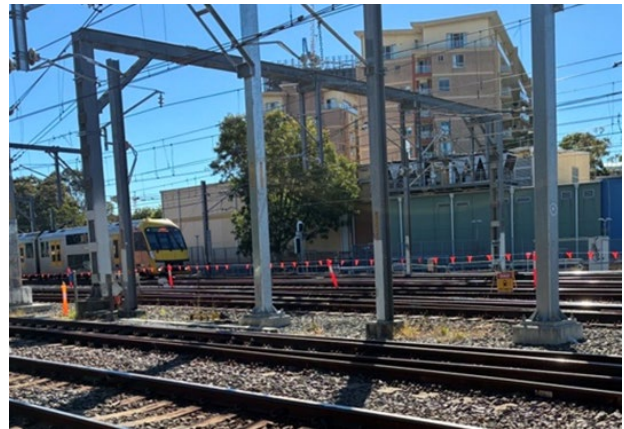
Photo 2: Placement of visual demarcation and signage at the location.
