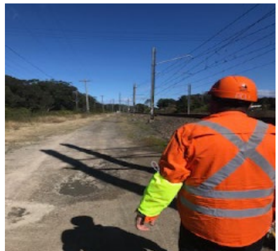
Image 2: Lookout in Up Cess looking for Down direction rail traffic
