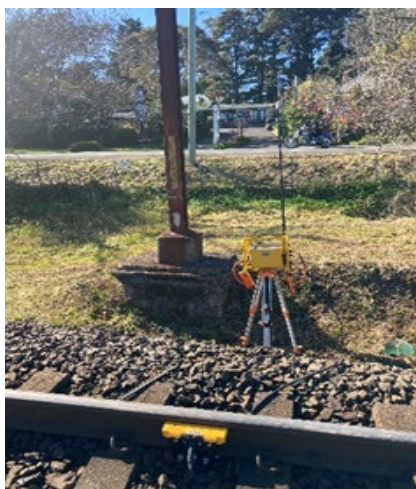
Image 1: Transmitter and sensor installation location
