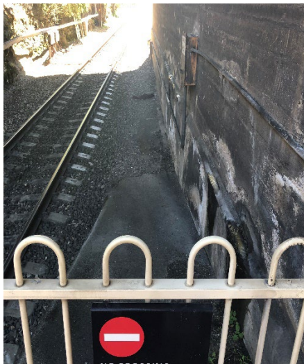
Image 3: Safe place for work at 96.6 Signal
