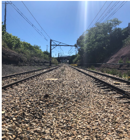
Image 1: View of Down direction Lookout at 155.515 KM in the 6 foot.
