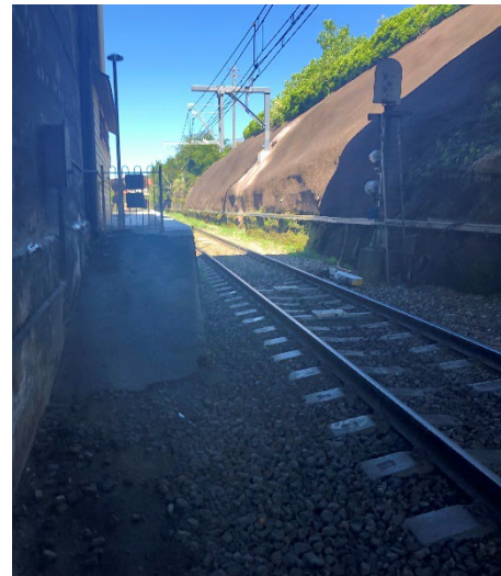
Image 4: Work Location at 96.6 Signal
