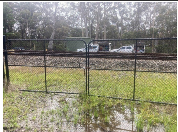
Image 2: Sensor access using access gate W00 116.782 U
