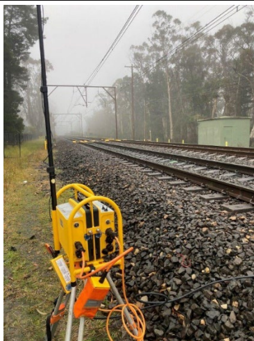
Image 1: Sensor and transmitter installation location
