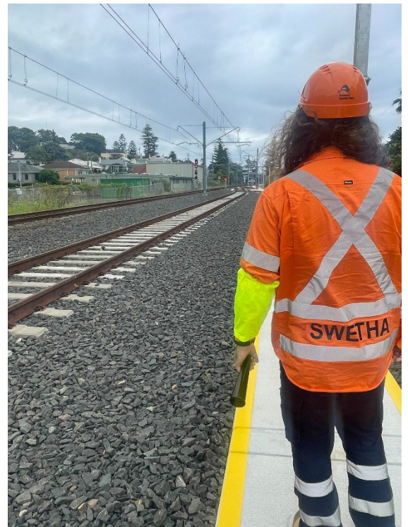
Image 2: Lookout view Towards Wollongong (Down Cess) – 119.550km
